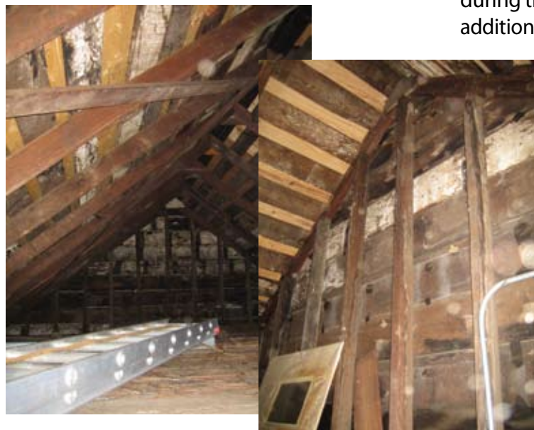
Dry rot in an attic with moisture problems
